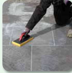
Level joints and wash surface until residue-free
