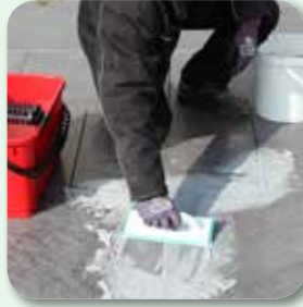
Work the mortar into the joints using the smoothing trowel
